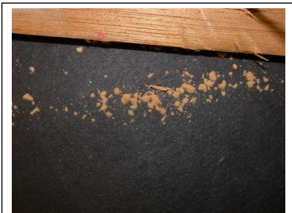
Fig. 4. Fine powder-like wood remains from powder post beetles. (Photograph University of Wisconsin – Madison, Department of Entomology)
