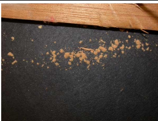
Fig. 4. Fine powder-like wood remains from powder post beetles. (Photograph University of Wisconsin – Madison, Department of Entomology)
